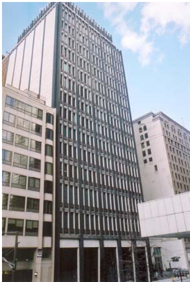
Adelaide Switching Centre (Bell Canada Centre) Toronto, Ontario
