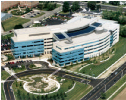
One Stone Road Guelph, Ontario Owner: The Ontario Government represented by the Ontario Realty Corporation Manager: SNC-Lavalin ProFac Inc.
