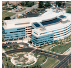
One Stone Road Guelph, Ontario Manager: SNC-Lavalin ProFac Inc. Owner: Ontario Government represented by the Ontario Realty Corporation (ORC)
