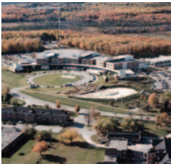
Lincoln M. Alexander Building Orillia, Ontario Manager: SNC-Lavalin ProFac Inc. Owner: Ontario Government represented by the Ontario Realty Corporation (ORC)
