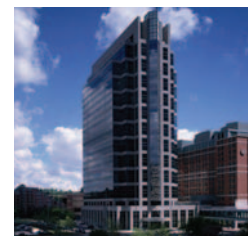
Ernst & Young Tower Calgary, Alberta Manager: Oxford Properties Group Inc. Owner: OMERS Realty Corporation, Oxford Properties, bcIMC (British Columbia Investment Management Corporation)
