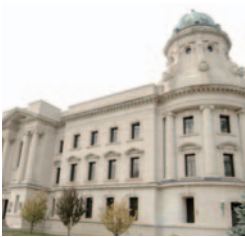
Manitoba Old Law Courts Building Winnipeg, Manitoba Manager: Manitoba Transportation and Government Services Operations Branch Owner: Province of Manitoba
