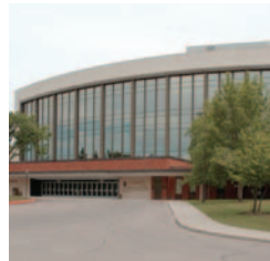
Southern Alberta Jubilee Auditorium Calgary, Alberta Manager: Alberta Infrastructure & Transportation Owner: Government of Alberta
